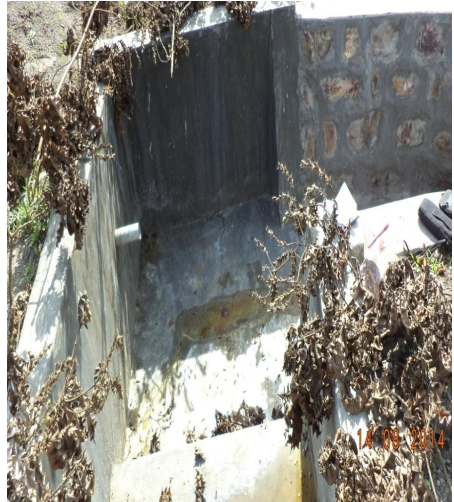
Protected source after construction at Gayaza Kasaali S/C
