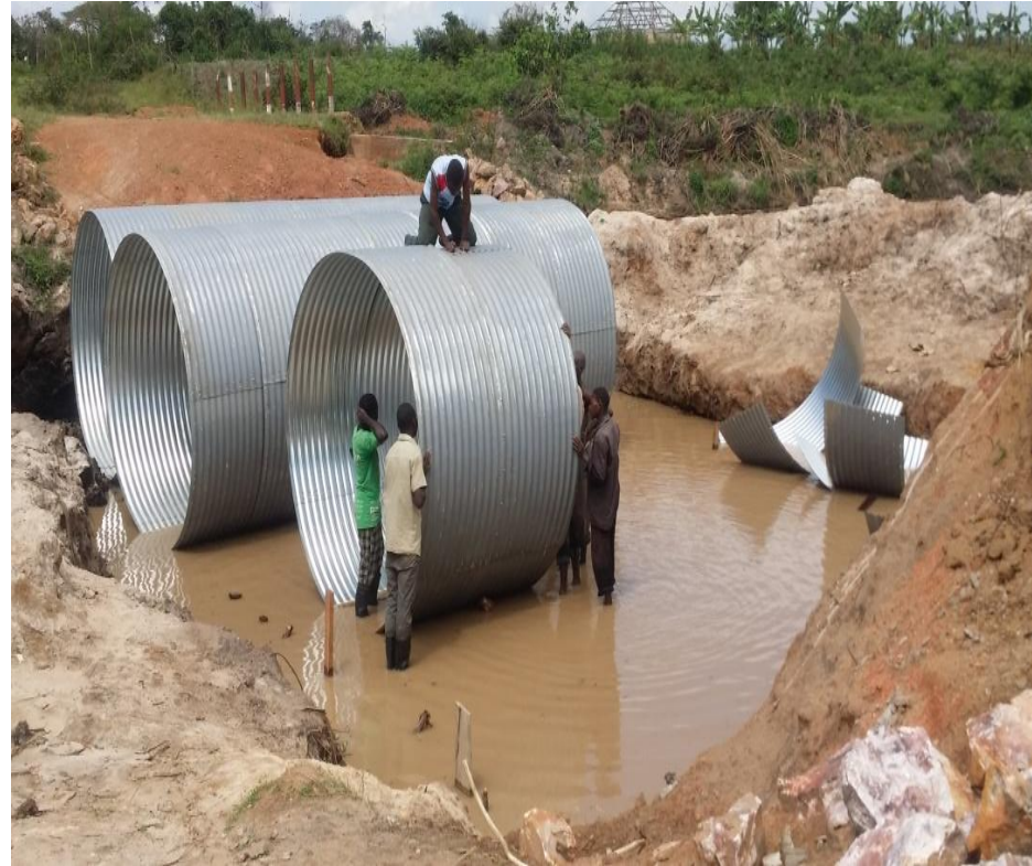
During installation of AMCO culverts
