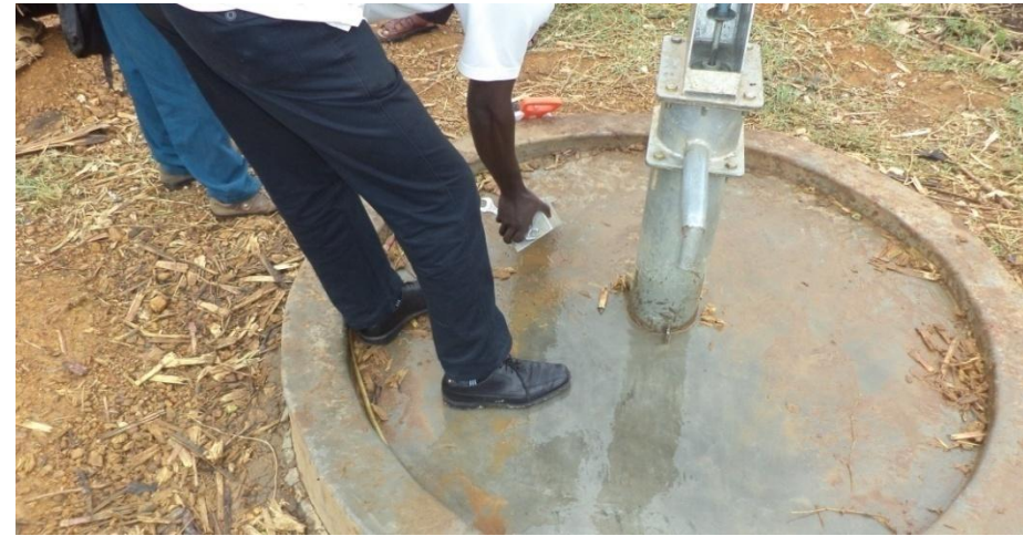
A poorly maintained shallow well, hence brake down
